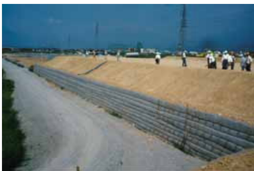
Fig.7 Completed pre-loading embankment.
