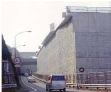
Fig.11 Completed wall with cantilever portion.
