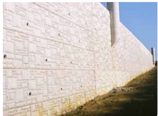
Fig.9 Foundation of pole combined with rigid aging.
